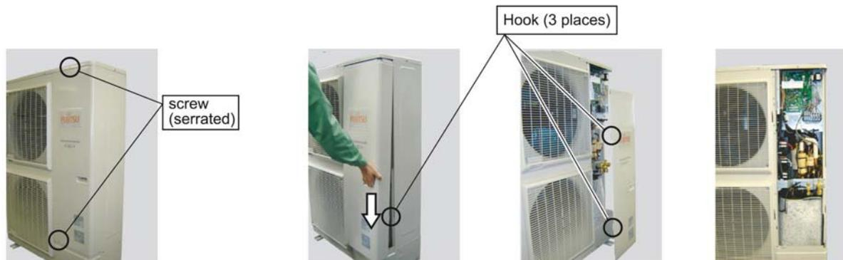
Remove the mounting screws.
