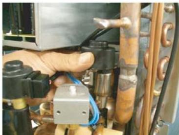
Remove the EEV coil by hand.
