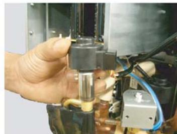
Remove the EEV coil by hand.
