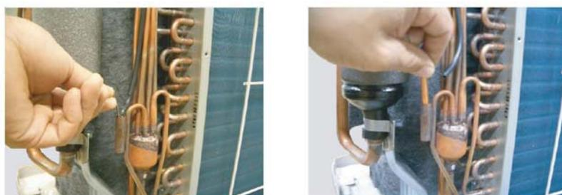
Remove the THERMISTOR SPRING. Remove the THERMISTOR.
