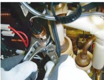
Remove the PRESSURE SENSOR
